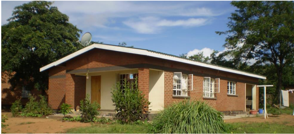
Figure 8 Staff House at Chilonga Health Center
